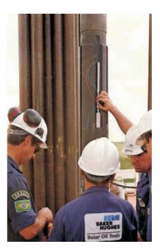
Installing and testing the world's first downhole electric wet-mateable connector system.
