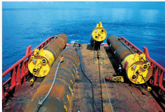
Delmar Systems' suction anchors for a preset mooring system are being deployed in the Gulf of Mexico.
