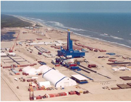
The Yastreb, designed and built by Parker Drilling, is drilling extended reach horizontal wells of approximately 36,000 ft to reach the northwestern flank of the Chayvo field offshore Sakhalin Island, making the wells among the longest in the world. The rig was sold to Exxon Neftegas Limited and is operated by Parker. Photo courtesy of Exxon Neftegas Limited.
