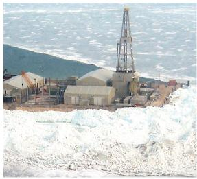
KCA DEUTAG's Rig T-47 has been drilling deep high pressure wells from an articifical island in the Caspian Sea since 2002. The rig was previously used on BP's Wytch Farm field drilling extended reach horizontal wells as long as 30,000 ft or longer. from the Piltun reservoir.
