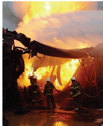
ALERT Well Control specialists cutting rig substructure and debris with a thermal lance to clear and access the well area. Photograph courtesy of ALERT Disaster Control.
