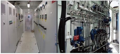
The reduced number of components installed on the permanent magnet motor winch makes the overall design simple and serviceable, which leads to less maintenance and easier troubleshooting. Above, compare the "engine room" on an electrical crane (left) with the "engine room" on a hydraulic crane.
