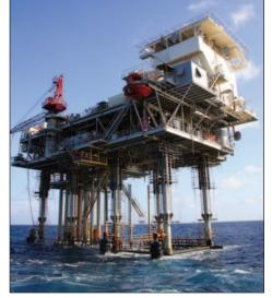
VERSABAR'S DECK RAISING system uses 32 synchronously controlled, 260-ton hydraulic cylinders to lift the platforms 14 ft each. The cylinders pin into lower padeyes welded to the existing legs and upper padeyes integral to the split extension sleeve. The 40 ½-in. diameter, 1 ½-in. wall extension sleeves capture the legs during the final leg cuts and, with rub rails, limit lateral movement during raising to 1/4 in.
