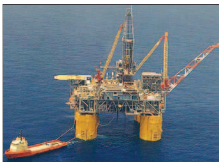
Figure 3 (above): Flow meter being functionally tested with the DAPC system during yard trial prior to deployment on deepwater GOM rig. Figure 4 (below): Mars TLP in deepwater GOM. Shell drilled a 50° re-entry well to 19,000-ft MD through depleted and abnormally pressured sands and unstable shales. They stabilized BHP and the wellbore by managing backpressure between 50-600 psi, reduced mud weight, continuously maintained ECD within 0.2 ppg tolerance, reduced overbalance from previous side-tracks, and eliminated losses using the Dynamic Annular Pressure Control system.
