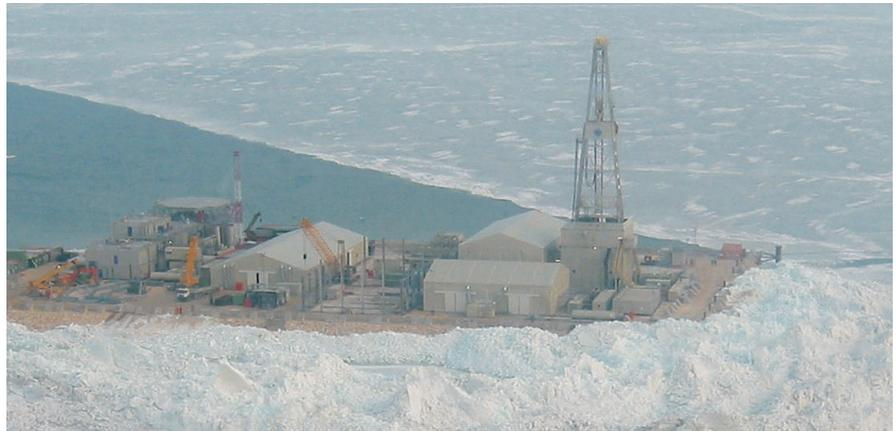
**KCA Deutag Rig T-47** is drilling for ENI-Agip on an artificial island in the Caspian Sea. The sloping sides of the island are designed to push the ice upward to generate rubble rather than allowing the ice to move across the island.
