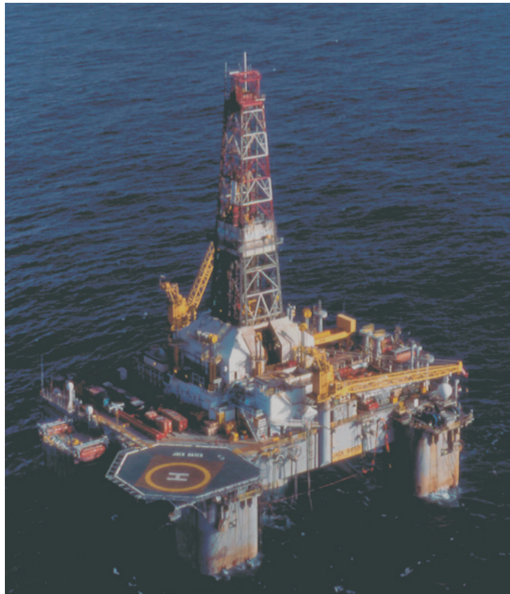
Transocean's semisubmersible Jack Bates is working for Shell offshore Ireland, with a well in the UK North Sea, also for Shell, scheduled following its current job.
