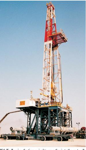
With Rig Buggies, the time rquired to move the rig to the next wellsite, usually about 50-100m away, is about 40 hours, although wellsite to wellsite would necessithere is scope for reducing this time to about 35 hours.
