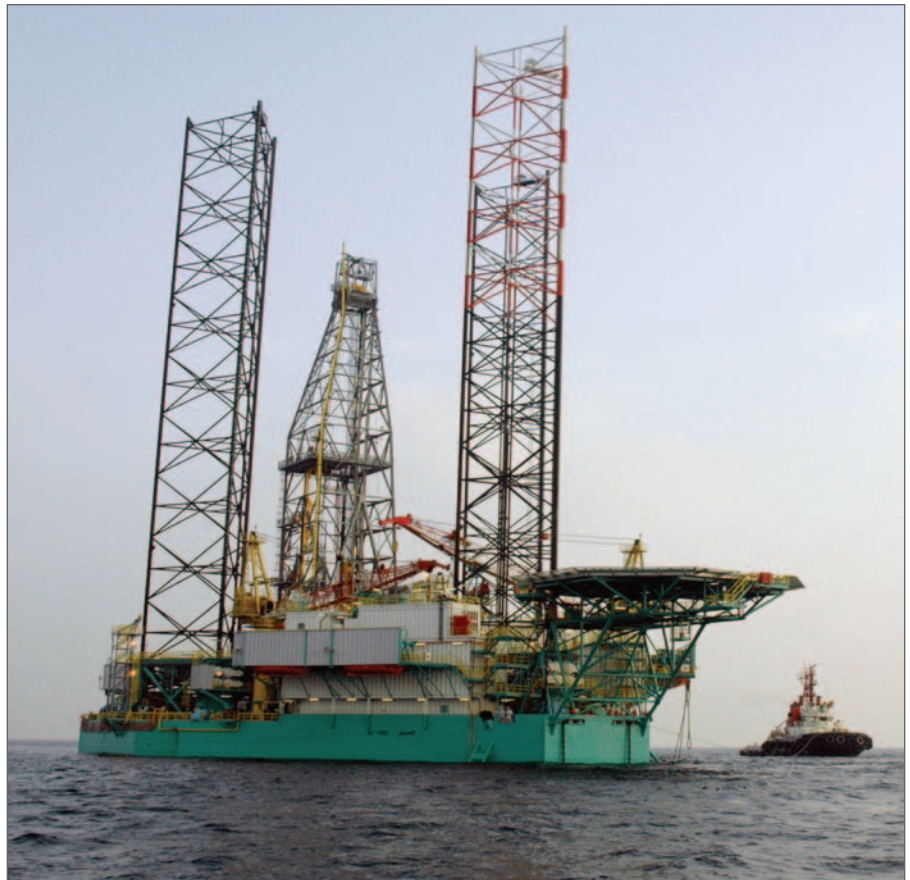
Abu Dhabi National Drilling Company currently has 16 land rigs and 10 jackups, including the jackup Al Hail (above), delivered in 2005. The company is now refurbishing and upgrading its jackup Al Bzoom.
