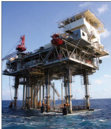
VERSABAR'S DECK RAISING system uses 32 synchronously controlled, 260-ton hydraulic cylinders to lift the platforms 14 ft each. The cylinders pin into lower padeyes welded to the existing legs and upper padeyes integral to the split extension sleeve. The 40 ½-in. diameter, 1 ½-in. wall extension sleeves capture the legs during the final leg cuts and, with rub rails, limit lateral movement during raising to ¼ in.
