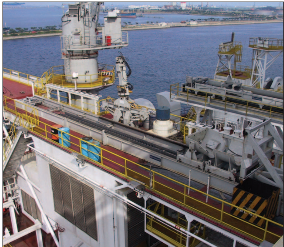
The Development Driller units' main catwalk has dedicated riser carts for transporting riser joints to and from the rig floor.
