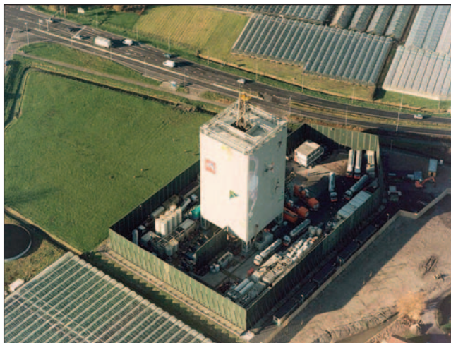
The cocoon — a steel structure with horizontal braces — is clad with sound insulation panels and can provide a sound reduction of about 10 dB.
