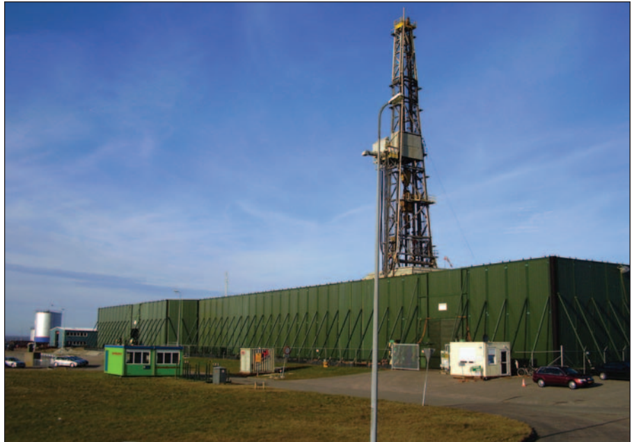
To minimize drilling noise at the source, sound walls are put up around the drill floor and fingerboard.
